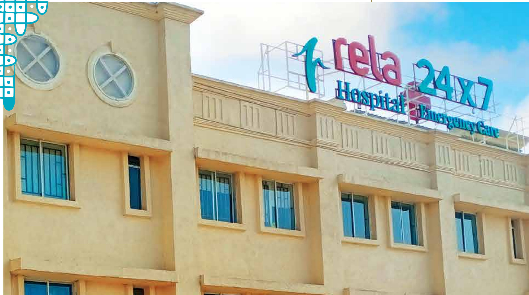
Actual image of RELA Hospital building
